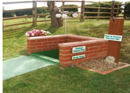
[Example of a chemical disposal point]
