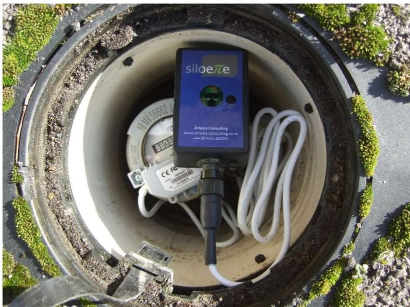
The logger records the flow through the meter at sub 1-second resolution. Once downloaded an algorithm is applied to the data to create a high-resolution flow trace of the flow into the property, as illustrated in Figure 4.
