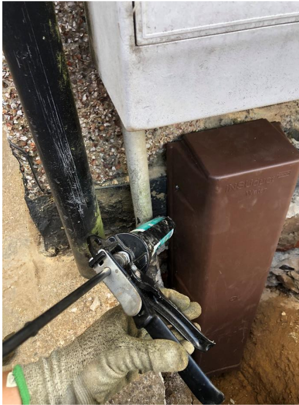
Boxing and insulation fitted and sealed.
