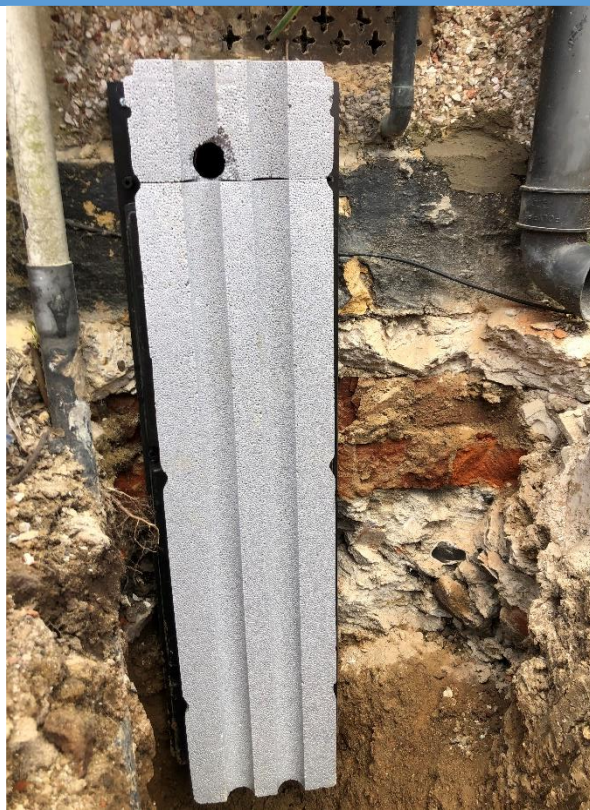
Back plate and insulation fitted
