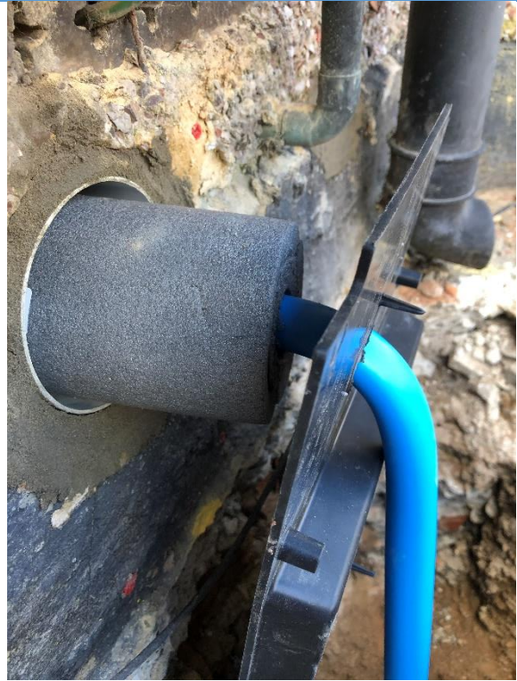
Insulation through duct 32mm thickness
