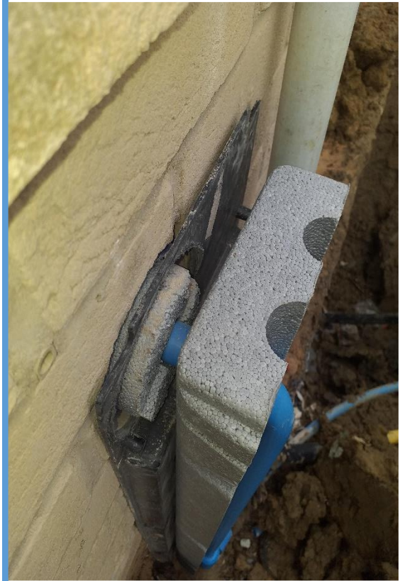
Photo of installation through wall.
