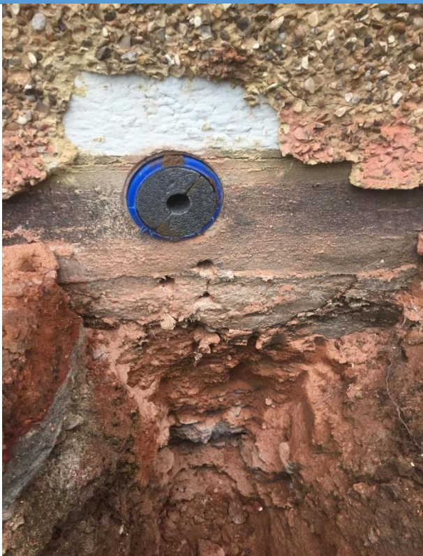
Installation of duct and insulation through wall.
