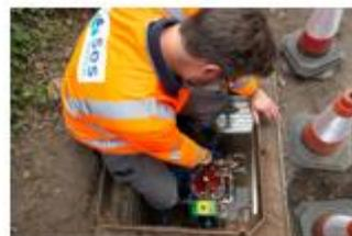
...Used smart technology to locate the position of burst water mains more quickly and accurately so they can repair them more quickly and reduce any interruptions to customers' water supplies
